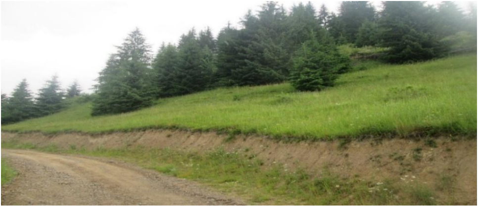
Figure 1. Fertile topsoil layer - v. thin
